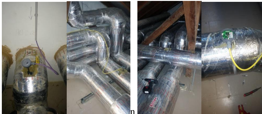
Fig. 12 The 4 air speed meters installed
