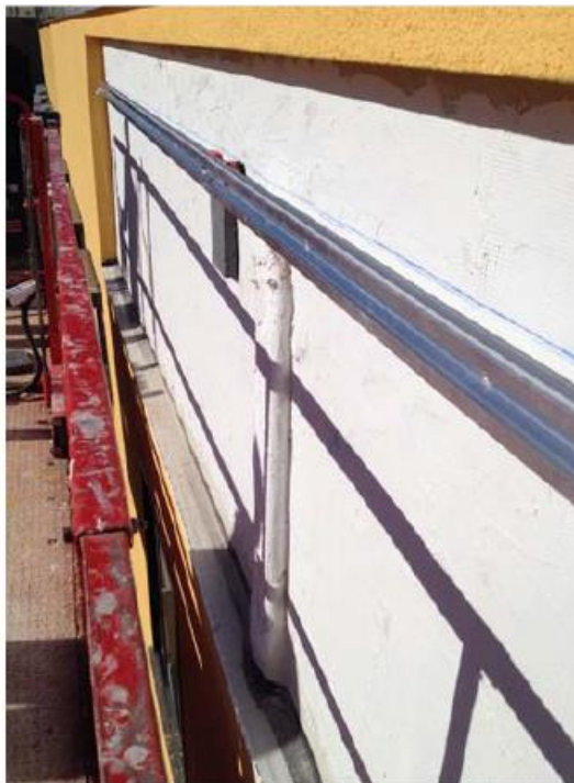
Figure 4. Photo after the installation on the first clipping profile
